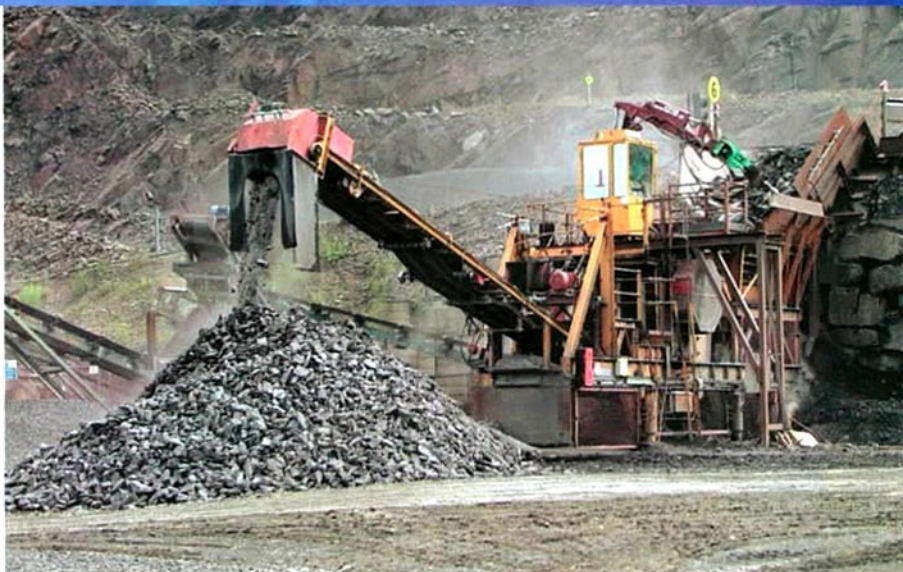
Energy-efficient technologies for electric motors are a practical solution for variable load equipment such as crushers and conveyors.
