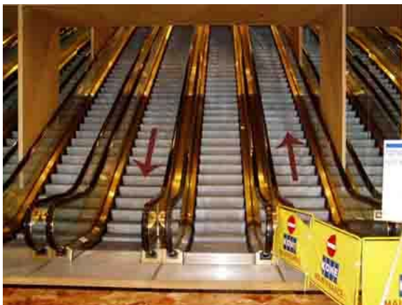
Figure 3. Test Load (“Up” and “Down” Escalator)
